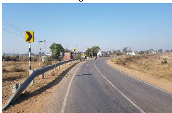
W Beam MCB at approaches at Km. 4+000
