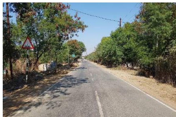
Pedestrian Crossing board at Km. 15+540
