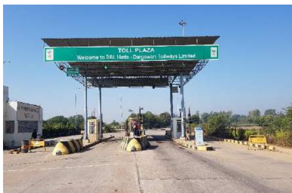
Toll Plaza at Km. 6+100
