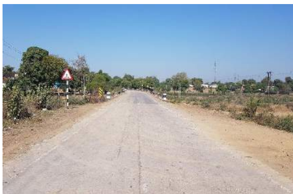
Pedestrian Crossing board at Km. 8+000
