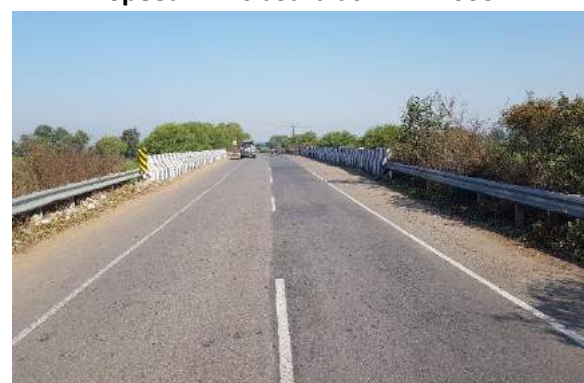
Safety at bridge approaches at Km. 4+250
