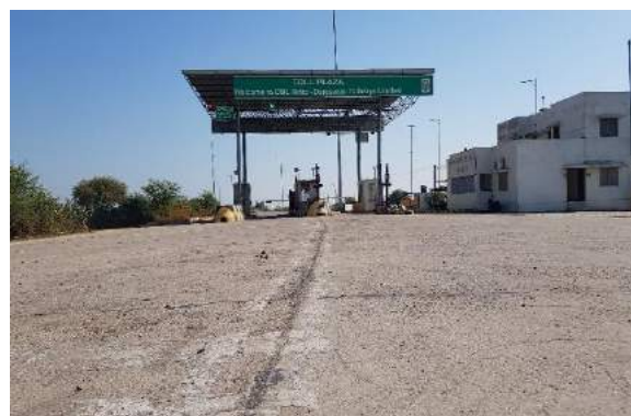
Toll Building at Km. 6+100
